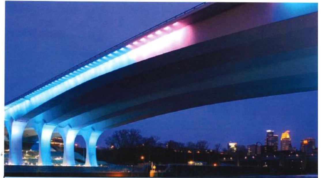
I-35W Bridge – Minneapolis (Blue/Purple LED Lighting)
